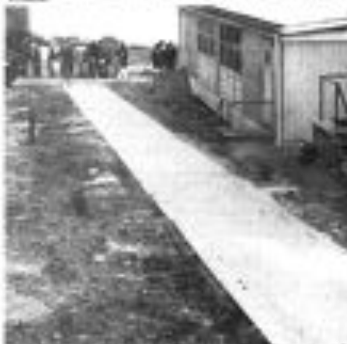
Newly constructed student walkway
