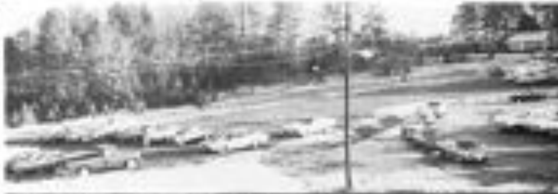
Duke Power Company is the gravel parking lot, which is being marked in.
